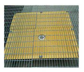
The drain pan attaches underneath 1" structural open grates in multi-level process areas by 8 anchor clips positioned on the outer rim of the pan as pictured above. The shower/eyewash station would be installed on top of grate above the drain pan. The drain in the center of the pan is a PVC slip joint with 3" ID and 4" OD. Field pipe installation to the center drain is a maximum 2" schedule 80 slip-in type pipe insertion depth of 1½".
